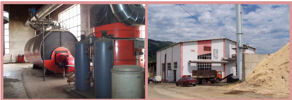
Thermal power plant operating on sawdust used to power a network of local heat in Vatra Dornei, Romania
