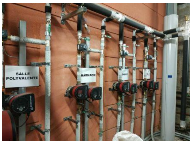
Network of the biomass heating plant
